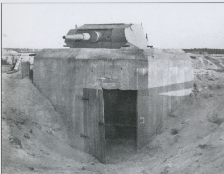
An example of a Pz.Kpfw.III panzerstellung at Hillersleben showing the rear armored access door.
