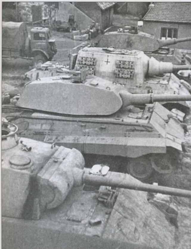
A US infantryman rushes by a knocked out Kingtiger near Weverousch, Germany on 27 March 1945. An internal explosion has blown off the turret roof.
