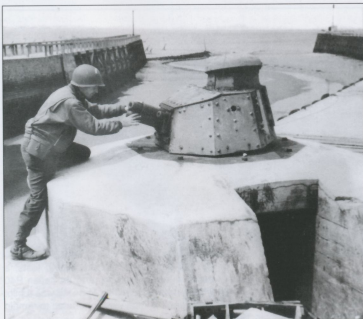
One of the more widely used turrets for coastal defense in Normandy was the old Renault FT turret like this example on a tobruk in the harbor of Grandcamps-les-Bains.
