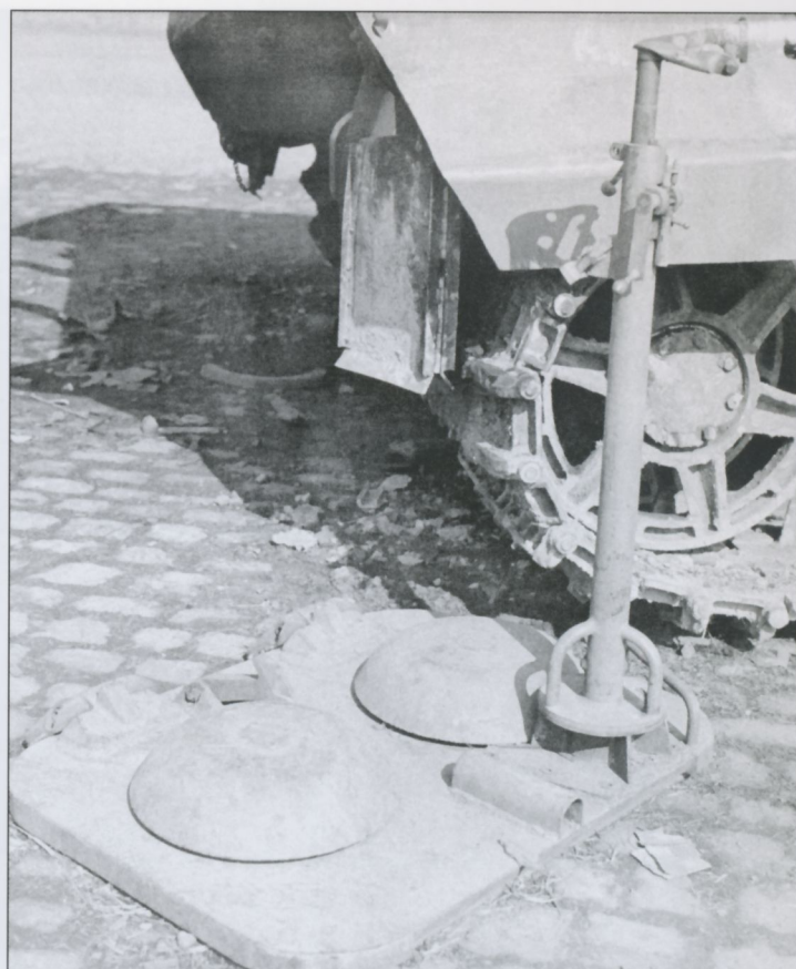
Technical intelligence teams inspecting one of the Jagdtigers of s.Pz.Jg.Abt.512 near Paderborn in April 1945 took some detail shots of its features. This is the rear engine deck hatch and shows the pintle mounting for a rear MG-42 anti-aircraft machine gun.
