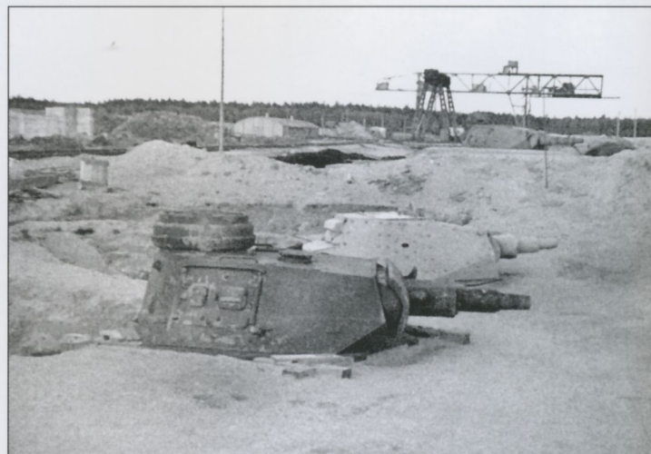
An interesting pair of turrets being used for panzerstellung tests, a short-barrel 7.5cm Pz.Kpfw.IV turret in the foreground, and an Italian P40 tank turret behind rearmed with the German 7.5cm gun. The P40 was a pilot for a program to rearm the Italian tank as the type was scheduled to remain in production in Italy in 1944.
