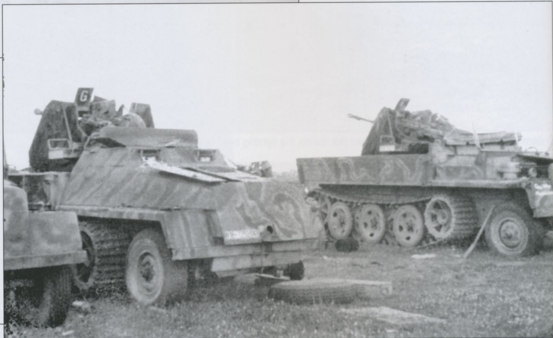
These two sWS halftracks with 3.7cm anti-aircraft guns were captured by the Polish 1st Armored Division in Germany in 1945. The nearer sWS is the type with the armored cab.
